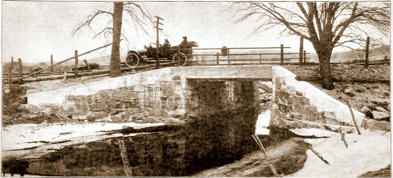
3A Bridge "B," "Turkey River." Re-inforced Concrete Floor. Roadway 20 foot wide. Capacity for Steam Road Roller.
