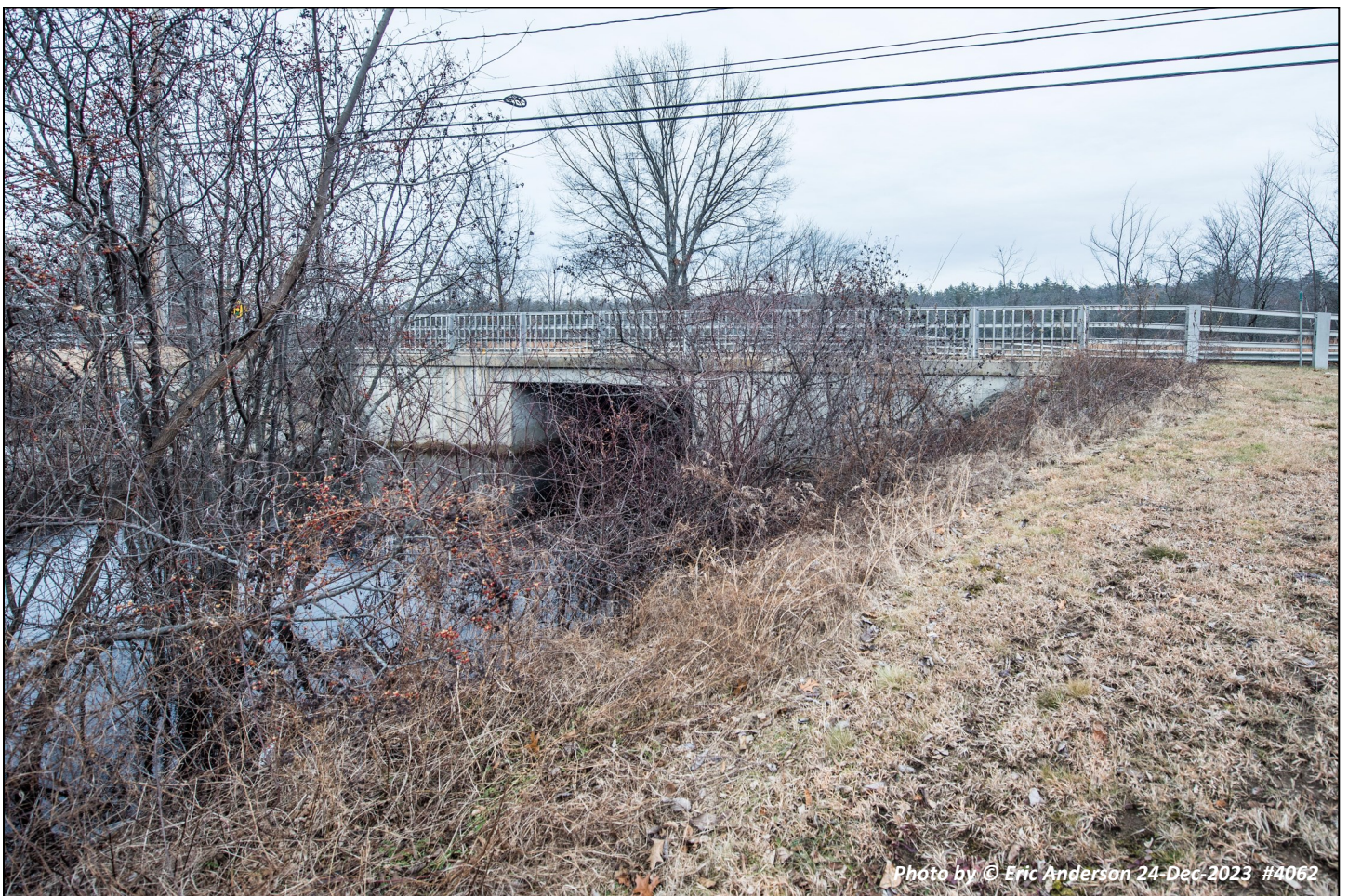
3A Bridge "B," "Turkey River." Re-inforced Concrete Floor. Roadway 20 foot wide. Capacity for Steam Road Roller.
