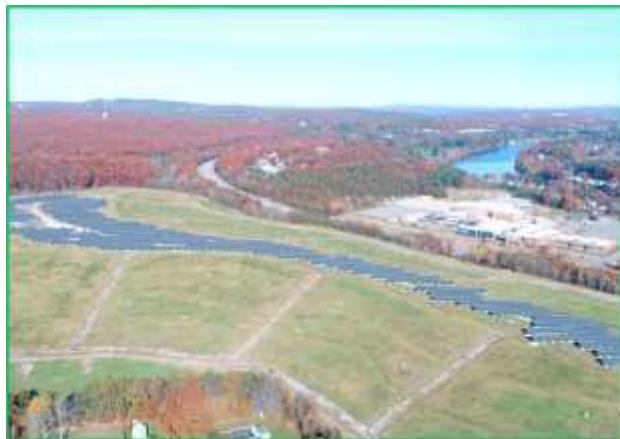
Kearsarge was awarded the right to develop, finance, construct and own this project through a competitive RFP issued by the City of Manchester. This project is New Hampshire's largest net metering project. The facility consists of a 3.3 MW DC ballasted ground-mount array located on the City's municipal capped landfill. The project's Commercial Operations date was December 2021. The City serves as the sole offtaker for the project.
