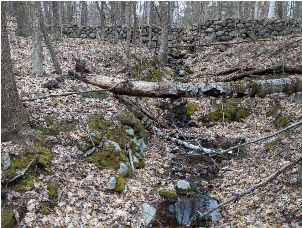
Photograph 16 Remains of stone-lined sluiceway along stream draining dam.
