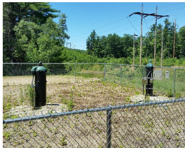
Figure 2-1 Existing gravel packed wells.
