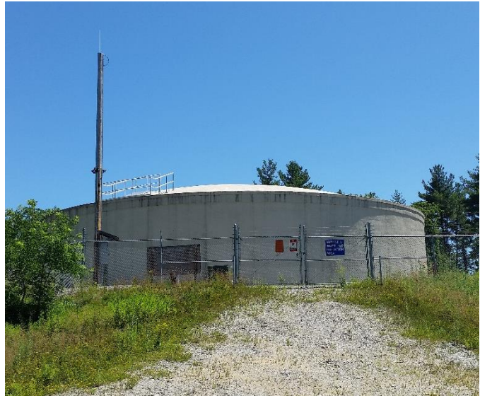
Figure 2-3 Existing atmospheric storage tank
