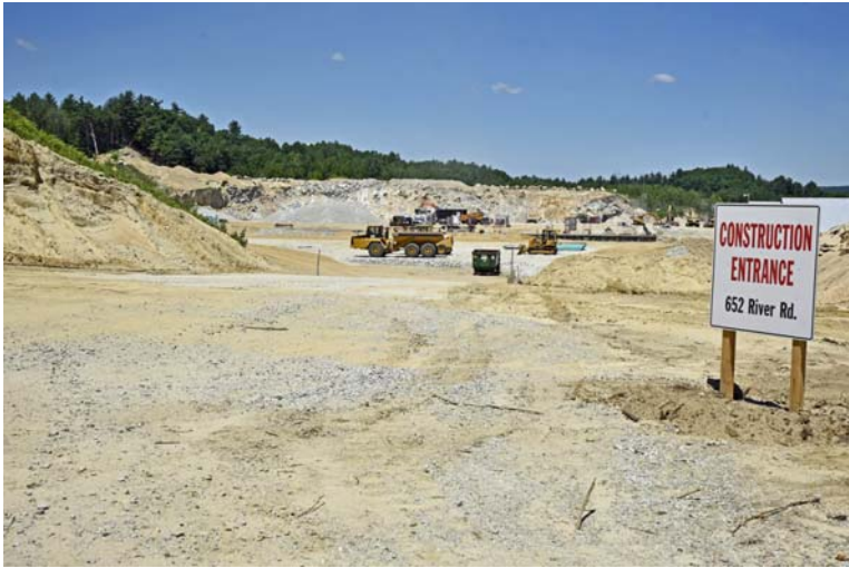
7/4/2018 Business Construction Project at 652 River Road, Bow, NH _DSC1020_edited-1-med7.jpg
