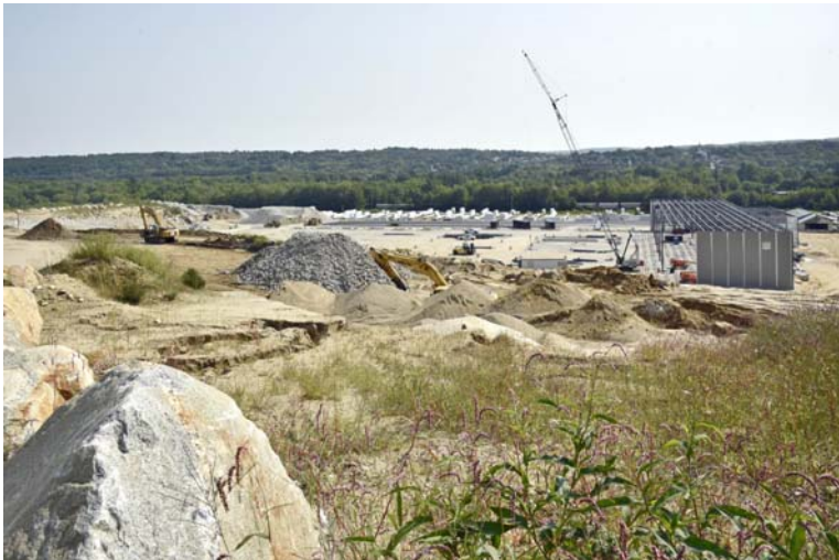
8/24/2018 Costal Storage Facility under construction _DSC1216_edited-1-med7.jpg
