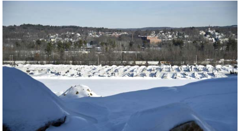
1/10/2018 Coastal Project - Site Work Underway _DSC9479_edited-1-med7.jpg
