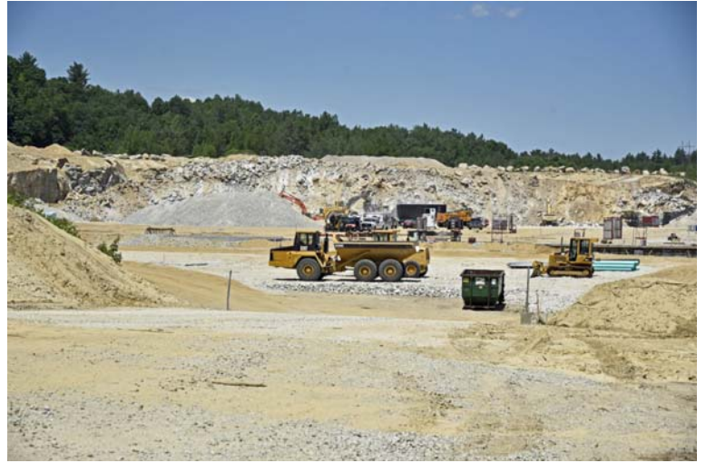
7/4/2018 Business Construction Project at 652 River Road, Bow, NH _DSC1022_edited-1-med7.jpg
