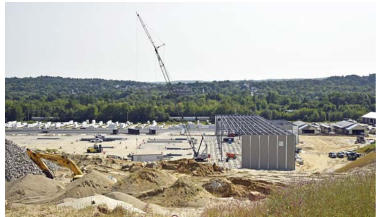
8/24/2018 New Coastal Facility under construction off of River Road _DSC1217_edited-1-med7.jpg
