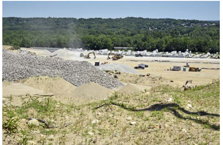
7/4/2018 Business Construction Project at 652 River Road, Bow, NH _DSC1027_edited-1-med7.jpg
