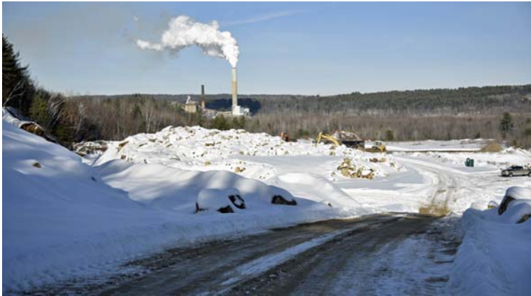
1/10/2018 Coastal Project - Site Work Underway _DSC9477_edited-1-med7.jpg
