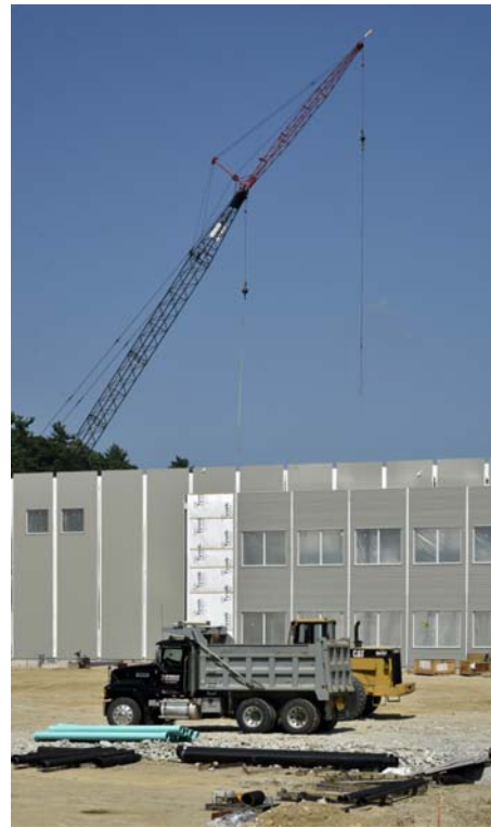
8/26/2018 Coastal Forest Productions Facility under con... _DSC1223_edited-1-med7.jpg
