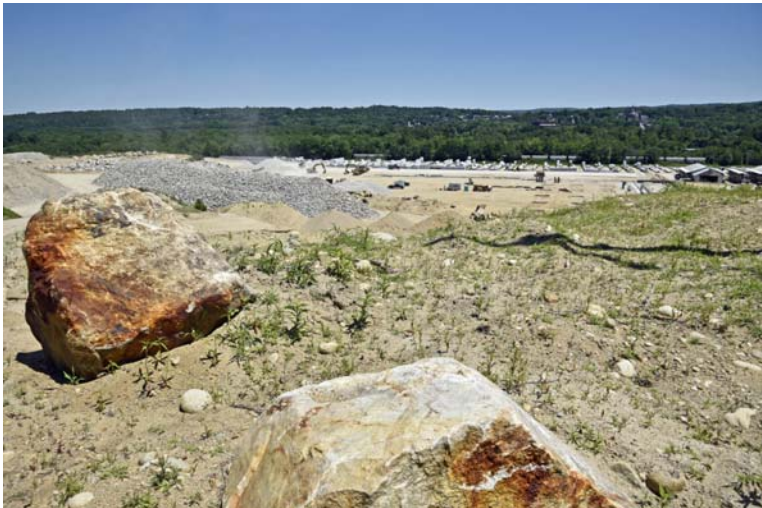
7/4/2018 Business Construction Project at 652 River Road, Bow, NH _DSC1025_edited-1-med7.jpg
