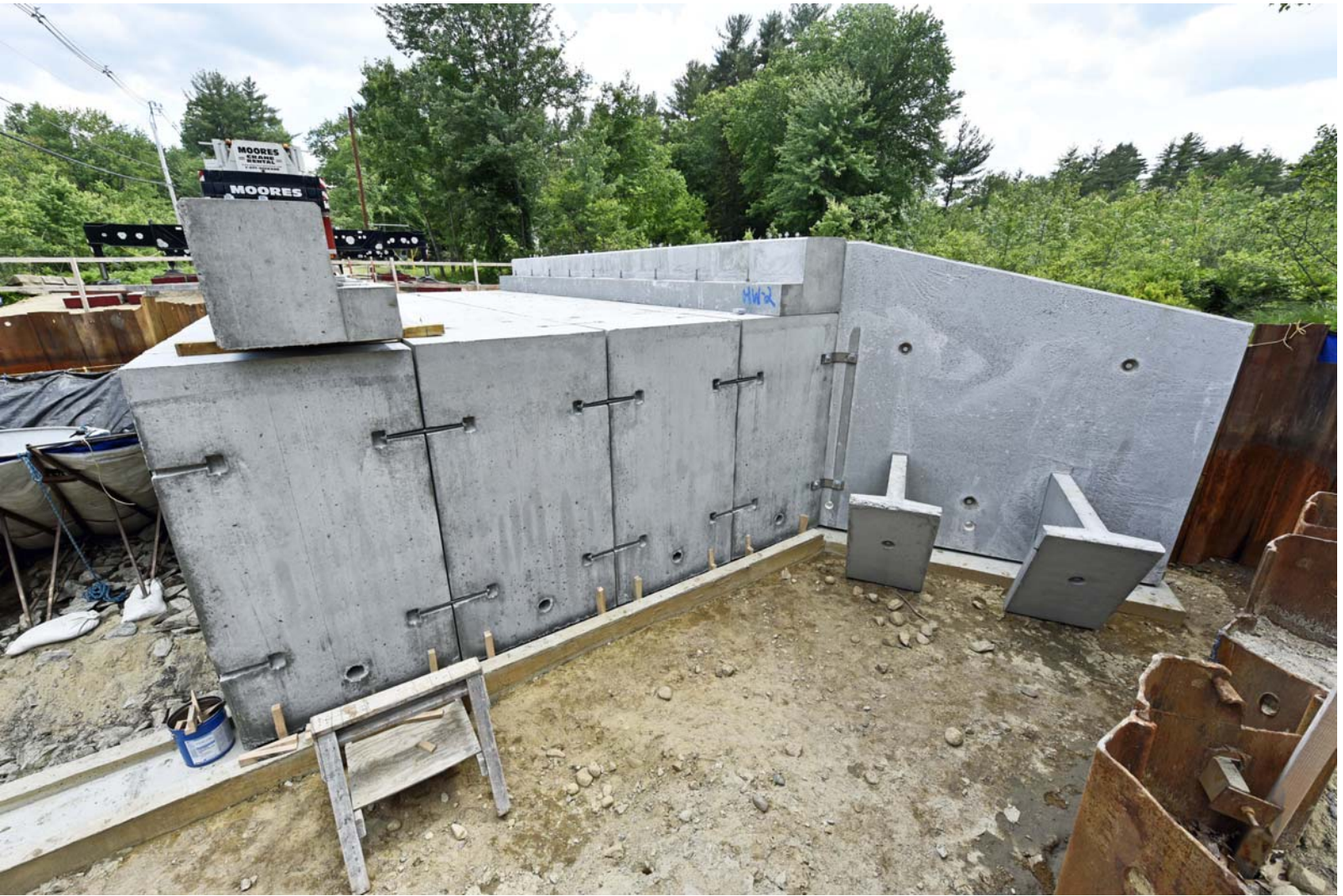
6/11/2018 Pre-cast segments bolted together _DSC0976_edited-1-med7.jpg
