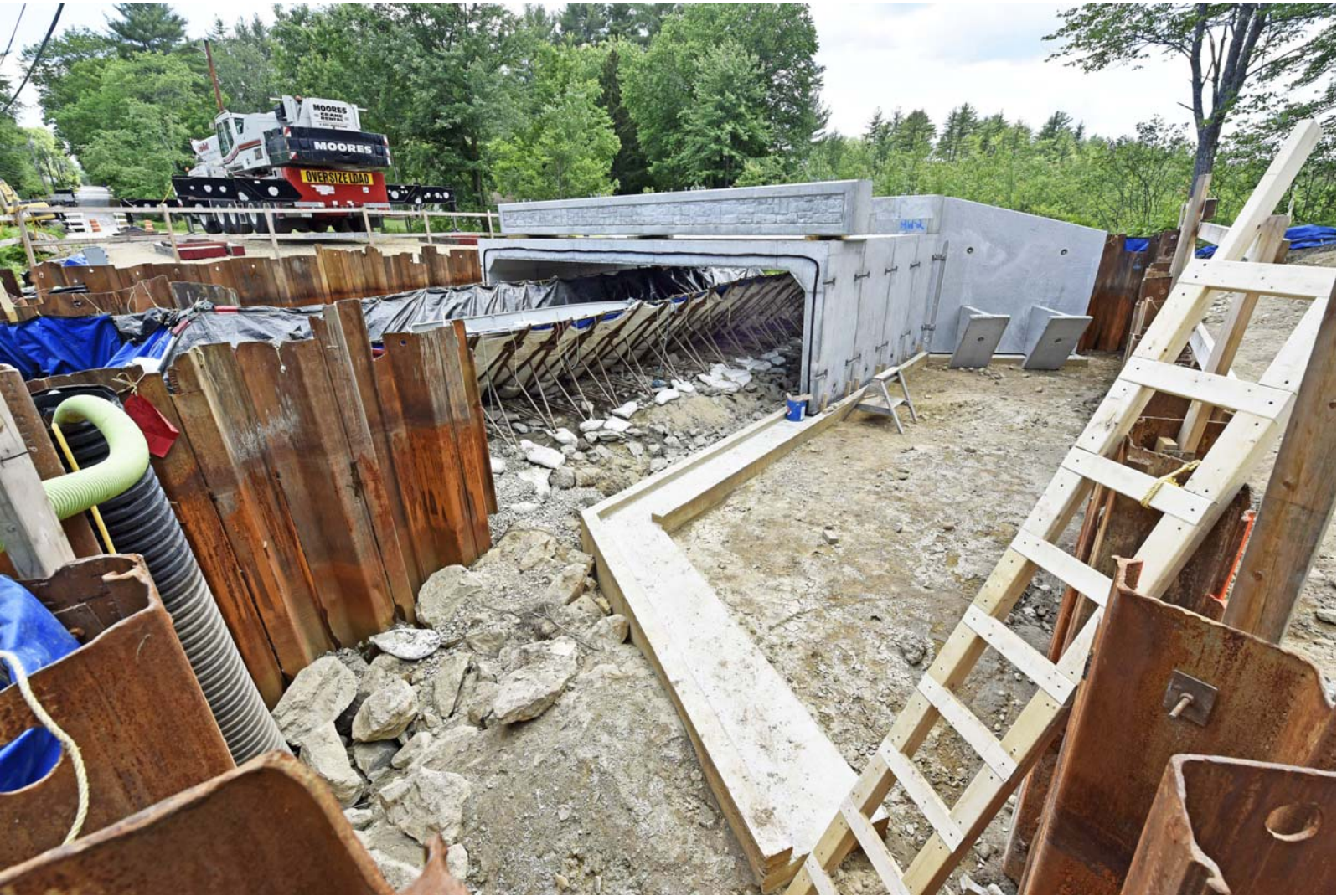
6/11/2018 Installing pre-cast concrete sections _DSC0979_edited-1-med7.jpg
