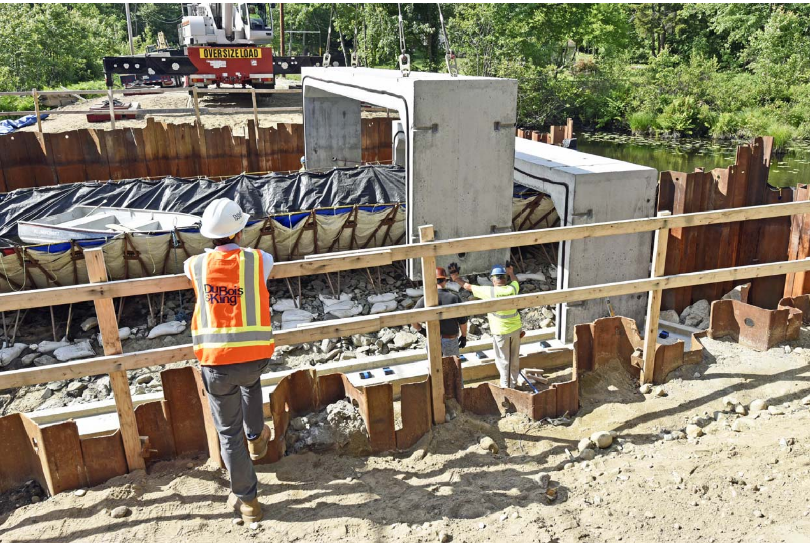
6/11/2018 Sections of the Birchdale Bridge begin going into place _DSC0877_edited-1-med7.jpg
