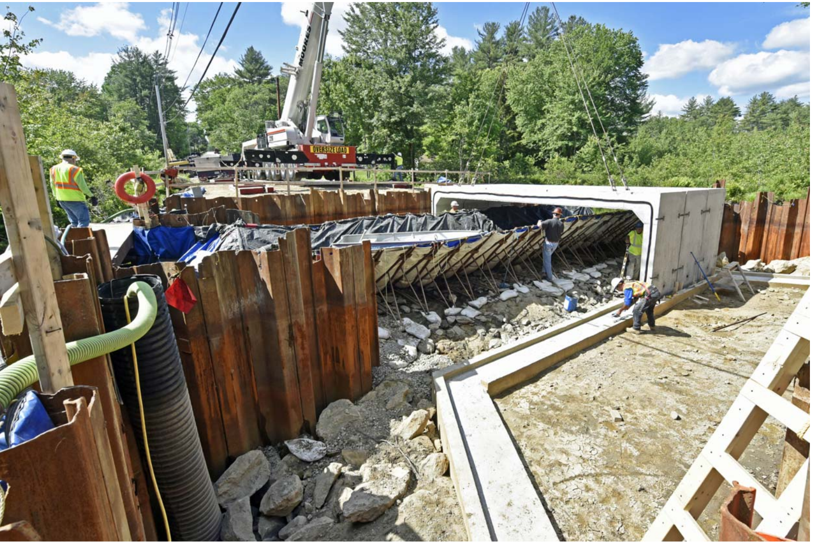
6/11/2018 Sections of the Birchdale Bridge begin going into place _DSC0944_edited-1-med7.jpg
