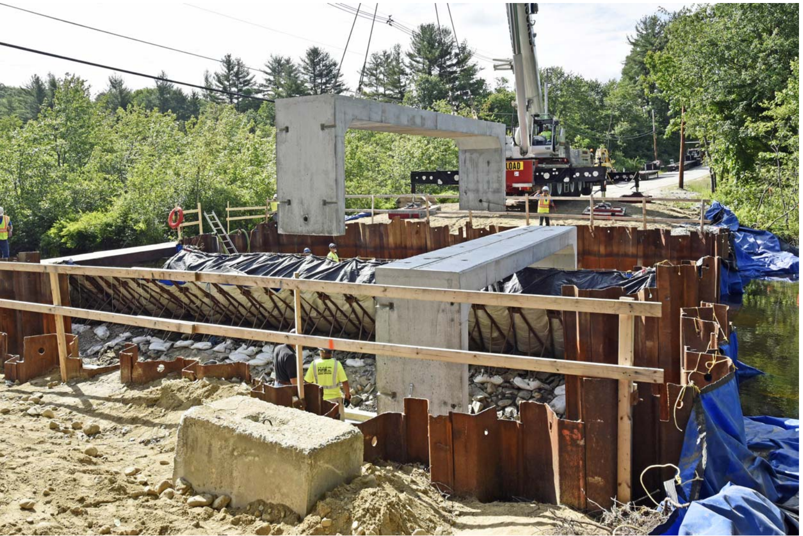
6/11/2018 Sections of the Birchdale Bridge begin going into place _DSC0874_edited-1-med7.jpg
