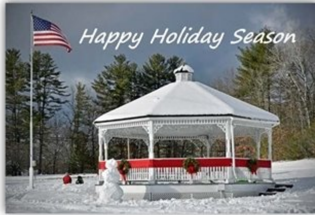
The Bow Gazebo—Logging Hill Road and Knox Road—Bow, NH—Built 2001
