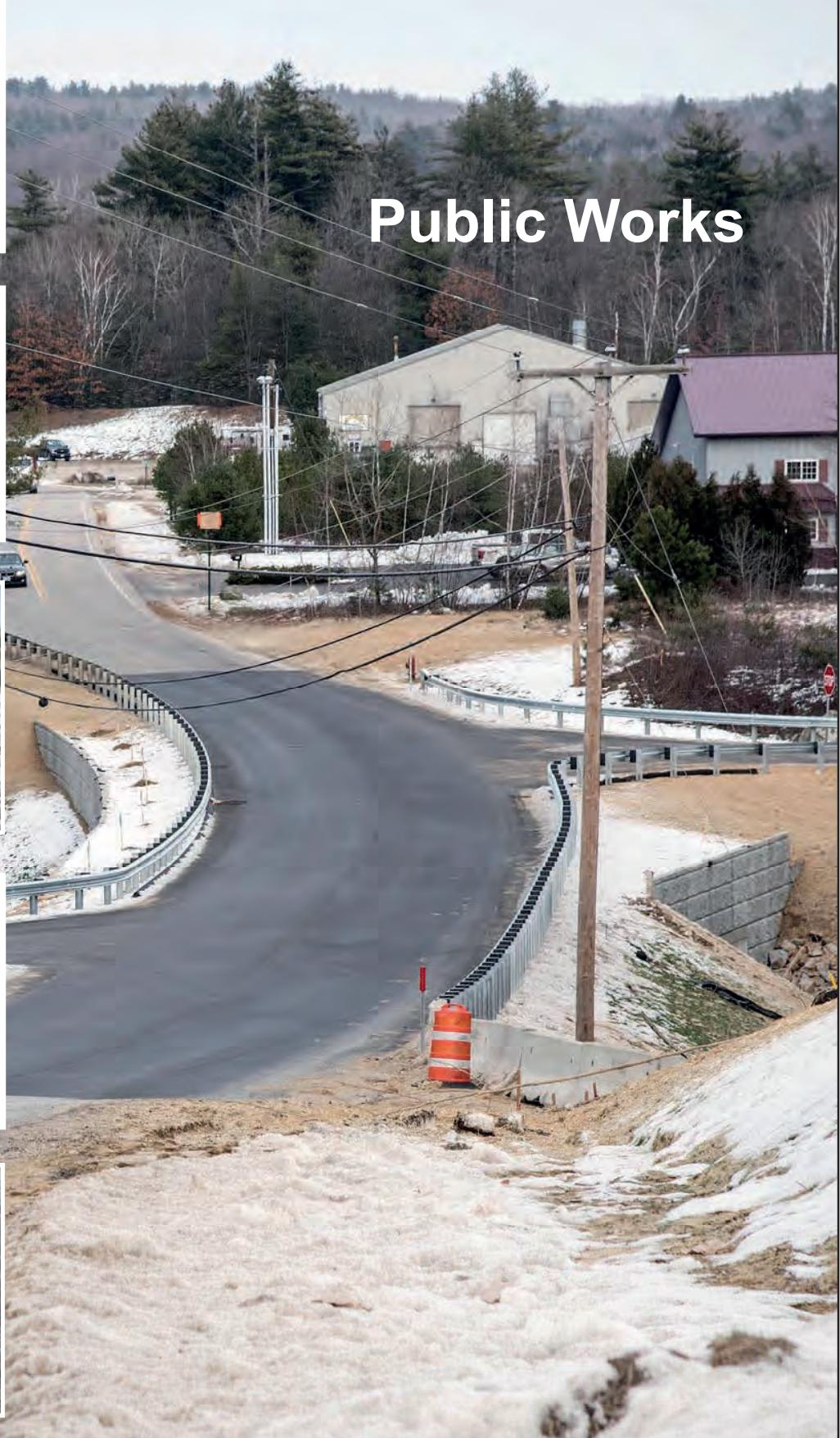
The Dunklee Road Bridge originally washed out during the flood of May 15, 2006. Because the replacement began to fail, it was again replaced in 2020
