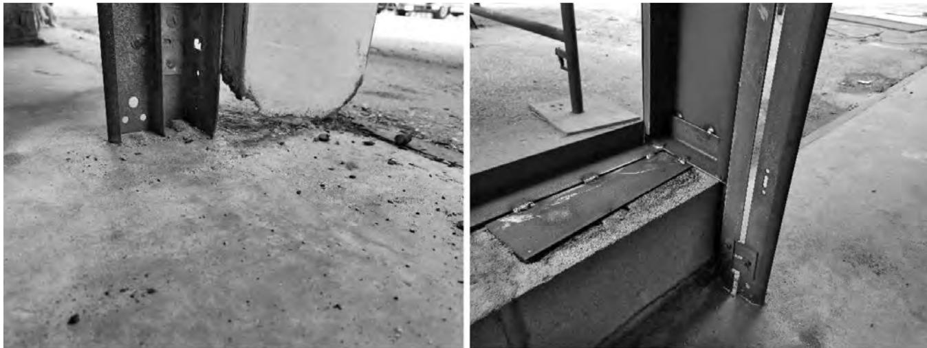
Several of the exterior wall partitions for the garage were rusted and no longer supporting exterior doors. The worst of these were fixed, and improved upon by the contractor and DPW staff.
